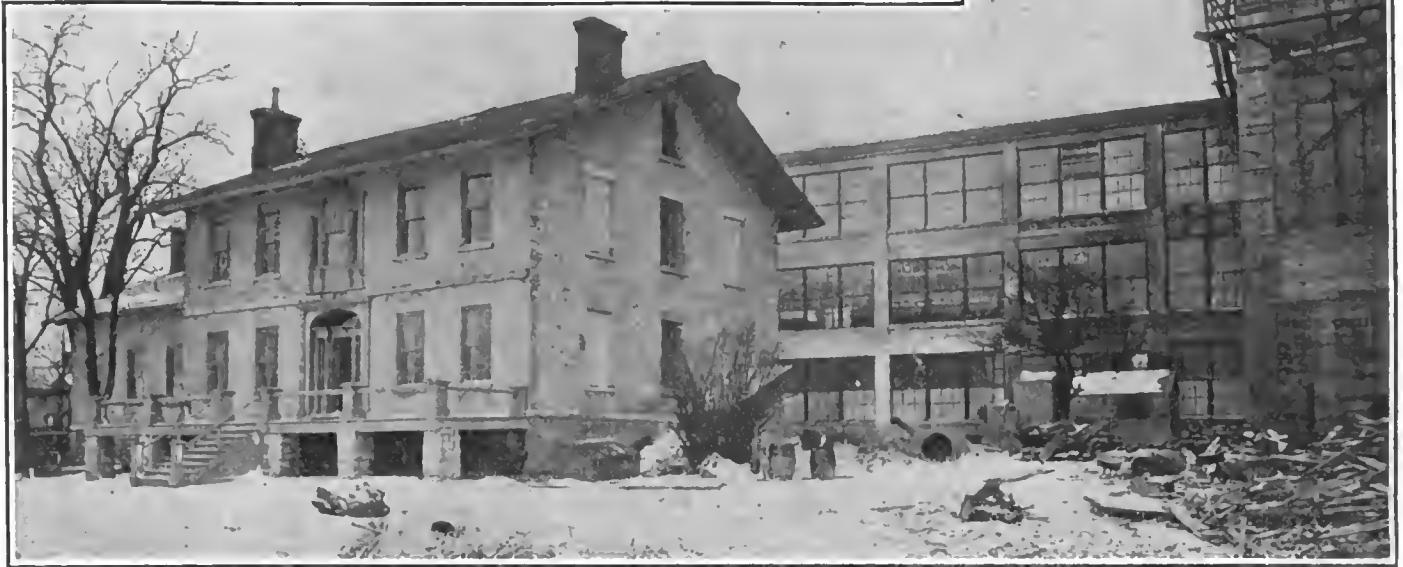
FRONT VIEW OF NEW THOMAS AUTOMOBILE FACTORY IN BUFFALO, SHOWING BOARD MOLD ON TOWER AT RIGHT FOR FORMING CONCRETE WALLS AND HISTORIC OLD MANSION IN CENTER REMODELED INSIDE FOR USE AS AN OFFICE.
